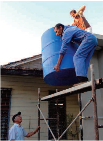
Lifting cistern into place
